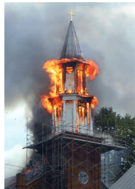
Figure 1 Steeple engulfed in flames before collapsing June 3, 2004
