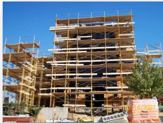
Construction of third church, October 14, 2007
