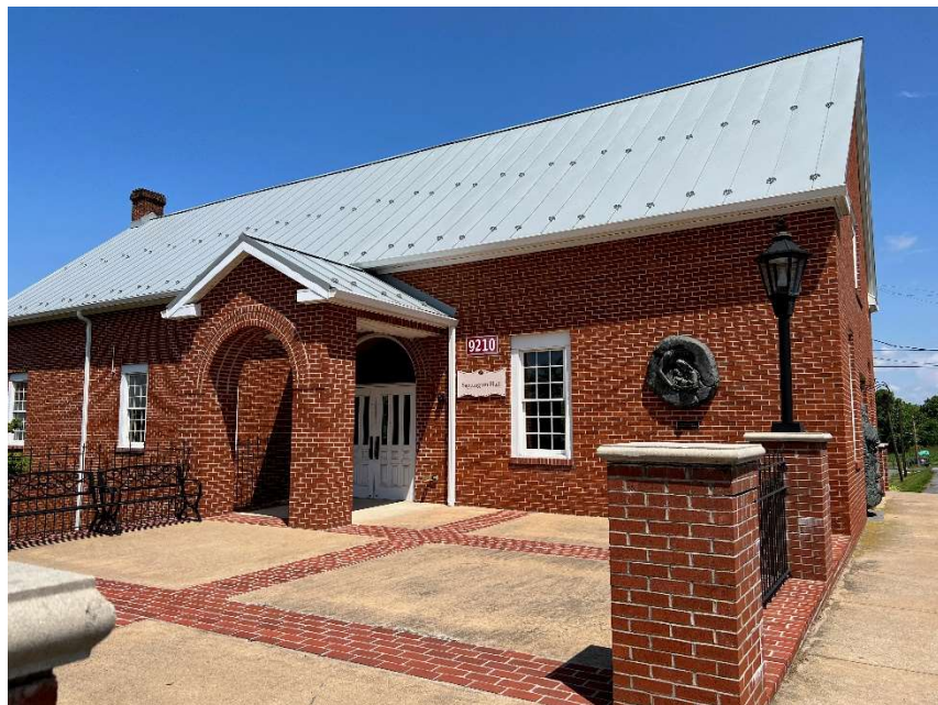
Sappington Hall after renovation, c. Summer 2023. (Courtesy, Ruth Riley, parishioner)
