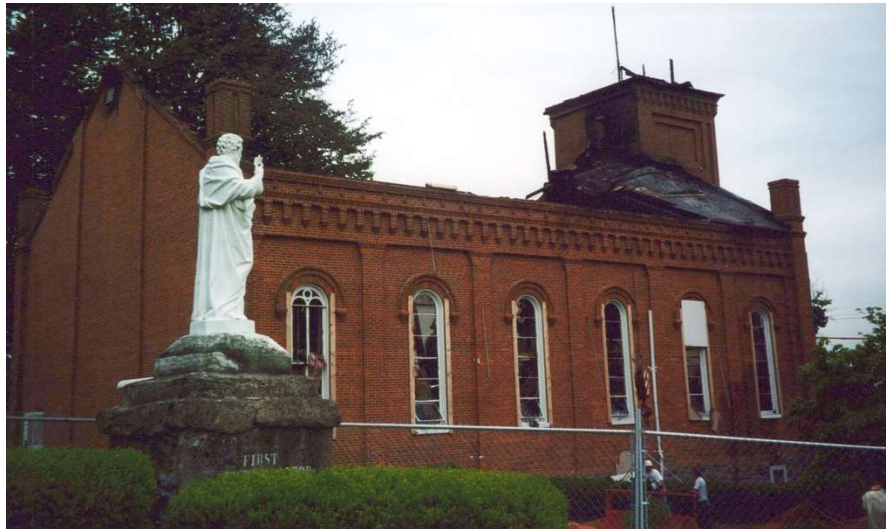
Aftermath of the fire, June 2004. (St. Peter's Archives)
