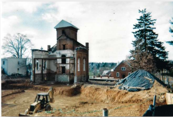
Excavating for construction of the third church c. early 2007
