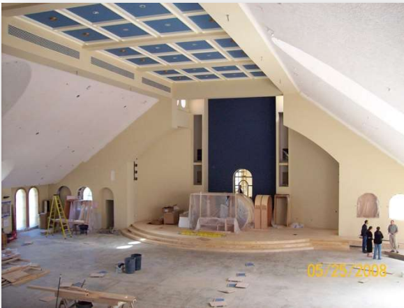
Sanctuary of third church under construction May 25, 2008
